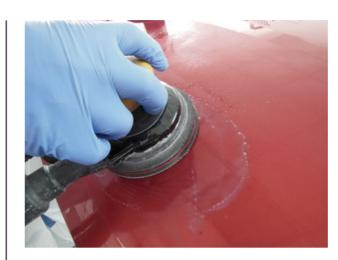
**3b. Large Area Inclusion Removal** For larger areas with more inclusions, use the P 1500 Film Disc on a 3 / 5mm DA Sander. Top Tip—use an interface DA pad to soften the abrasion.
